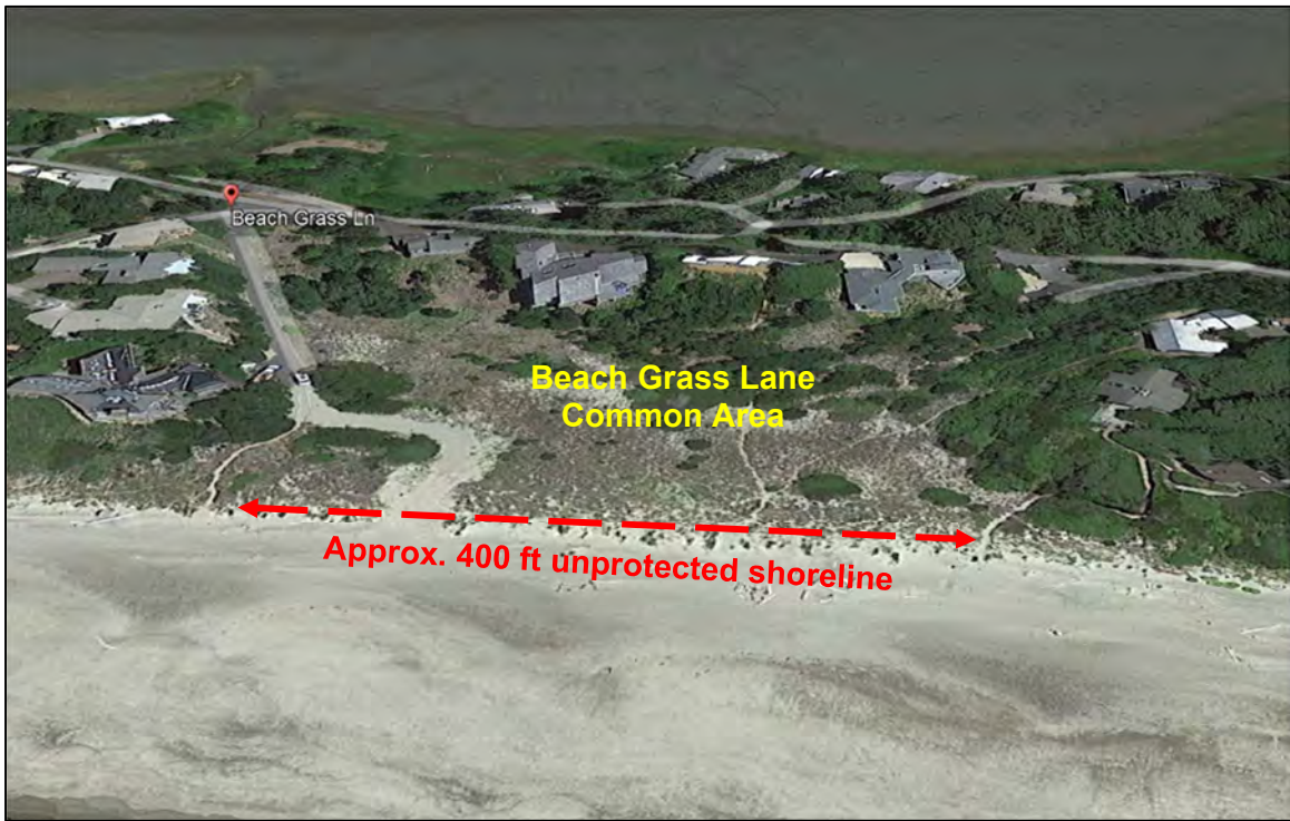
Figure 3: Google Earth image of the approximately 400 linear feet of unprotected beach frontage (imagery date: July 13, 2022)
