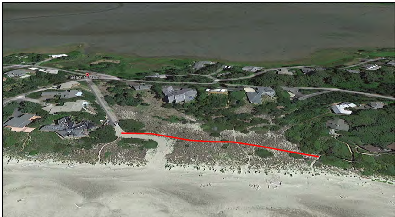
Figure 4: The extent of the erosion observed on February 9, 2024, as shown by the red line. (Google Earth imagery date: July 13, 2022)
