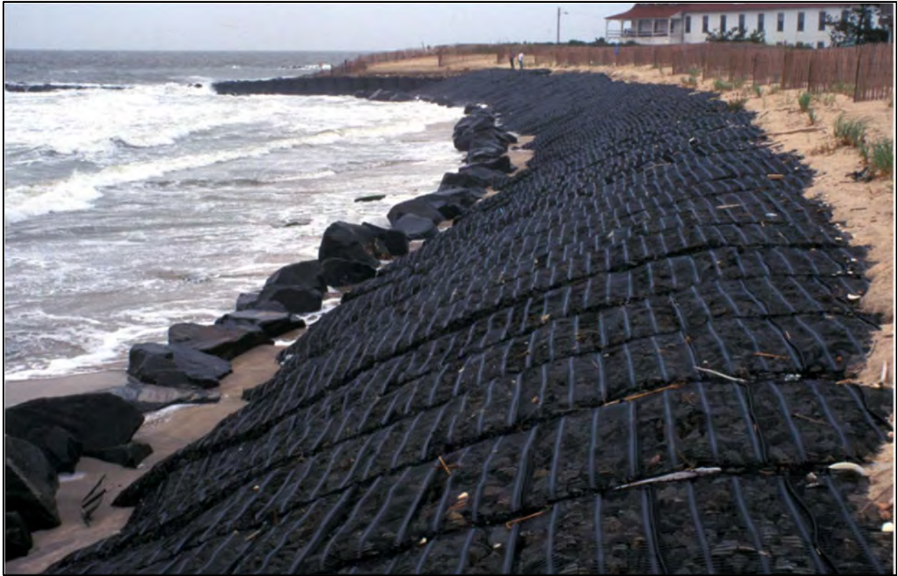
Figure 10: Example of engineered geosynthetic mattress system (Hughes, S.A., “Uses for Marine Mattresses in Coastal Engineering”, February 2006, ERDC/CHL CHETN-III-72, U.S. Army Corps of Engineers).
