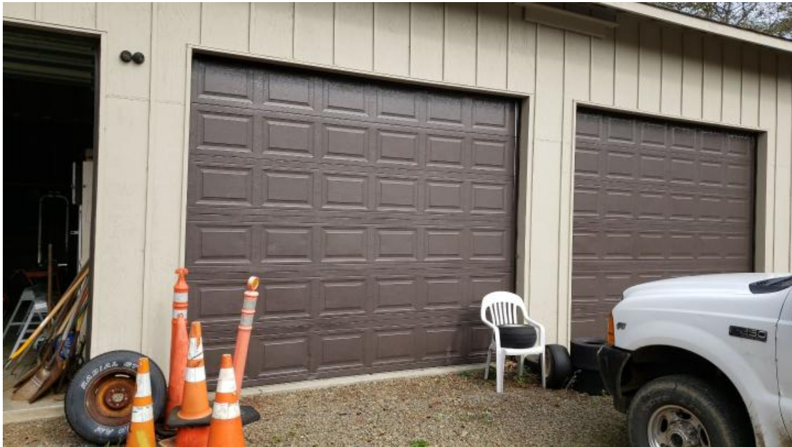
Building Exterior - Garage Door, 9'
