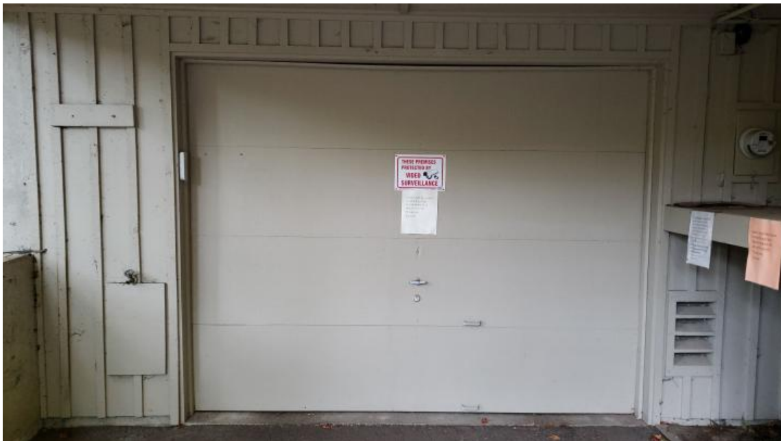
Building Exterior - Garage Door, 9'
