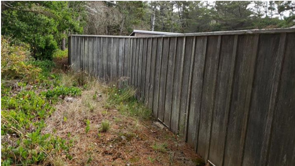
General Site - Fence, Wood @ Rec. Bldg
