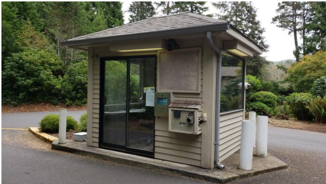
Building Exterior - Windows & Sliding Glass Doors
