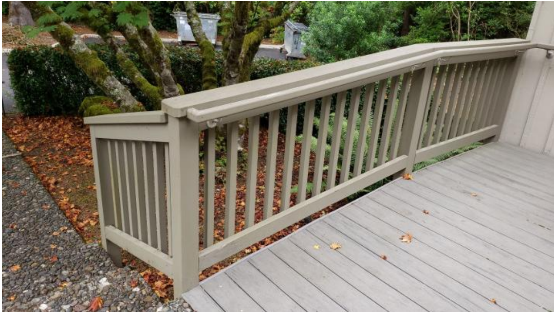
Building Exterior - Deck Surface, Wood Decking [Paint]
