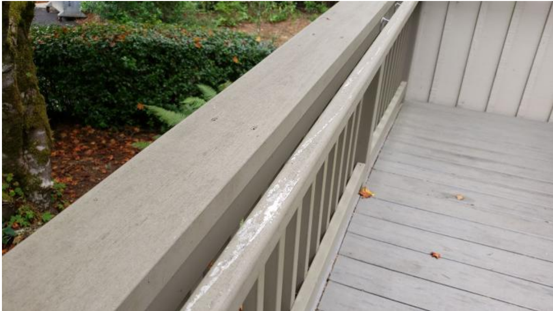
Building Exterior - Deck Guardrail, Wood
