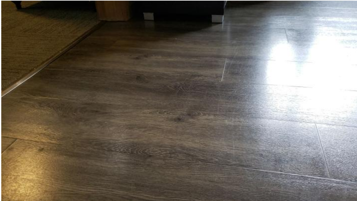
Building Interior - Flooring, Vinyl
